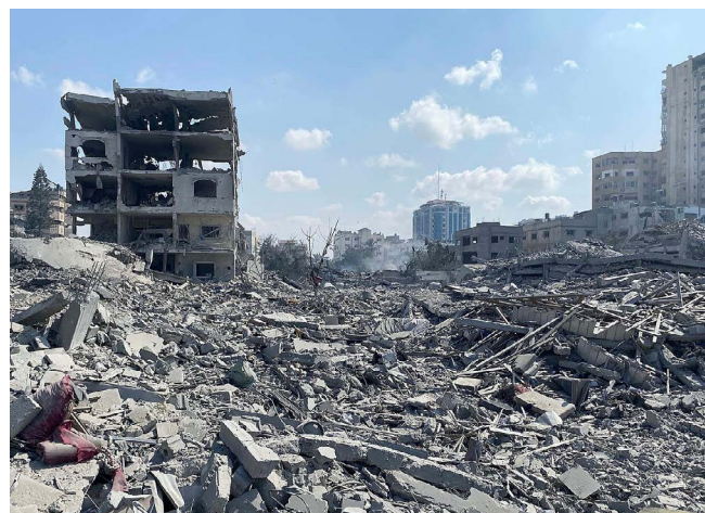
Damage following an Israeli airstrike in Gaza City on October 9, 2023
